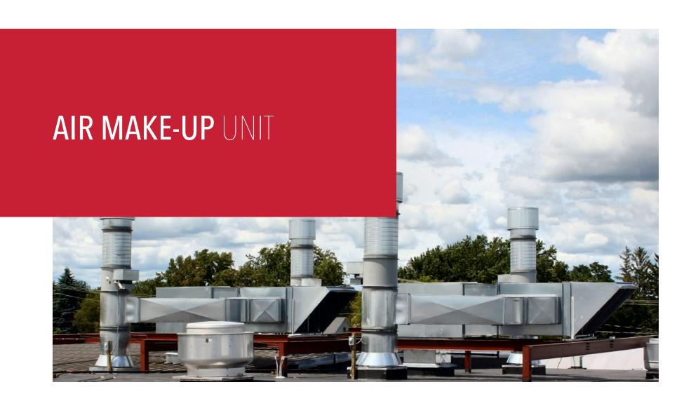
GFS' direct gas-fired air make-up units (AMU) provide an economical source of replacement air. By continually replacing contaminated booth air with fresh, heated outdoor air, AMUs maintain a constant air temperature regardless of the air temperature outside your building. This allows for balanced building pressure and proper comfort levels.
